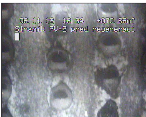
Detail perforace v hloubce 70,68 m
