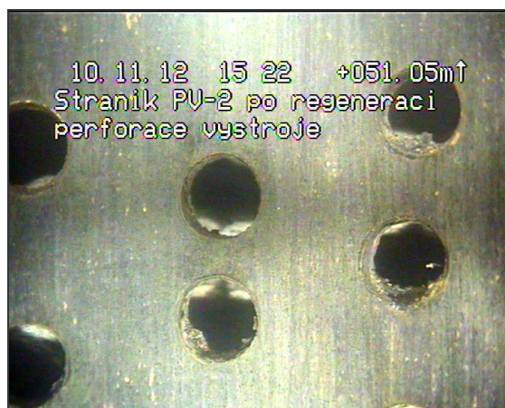
Detail perforace v hloubce 51,05 m
